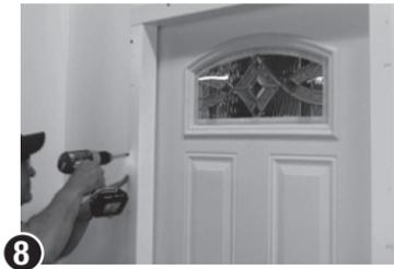
**8** Secure the header closure trim and jamb closure trim near the top corners. Then install the remaining screws.
