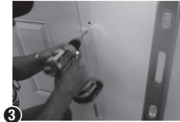
**3** Install screws in the hinge jamb, start at top, checking for plumb as you work to bottom.
