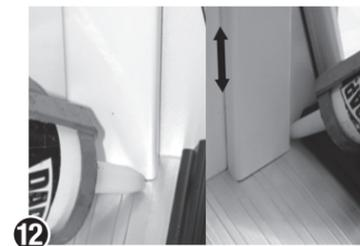
**12** Allow caulk to set before reinserting weatherstrip. Caulk outside sill and closure trim to floor. For exterior, caulk frame to closure trim at jambs & header (as arrow indicates).
