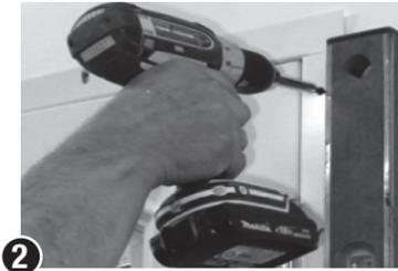
**2** Use a level to plumb hinge jamb. Secure near top corner with a drywall screw.
