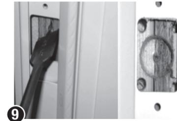
**9** Prepare stud for deadbolt clearance. Bore a 7/8"-1" hole to a depth of 1" from face of frame. Drill a 3/8" diameter hole at corners - 1" from face of frame.
