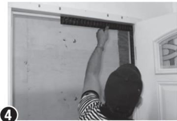
**4** Remove prehang clip and open door. Square header to hinge jamb. Install drywall screw in center of header.
