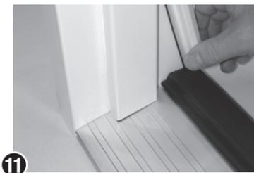
**11** Pull weatherstrip out of the kerf near sill to allow room for caulking. Install sill extender if required.
