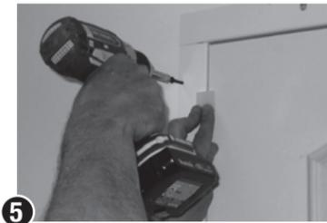
**5** Close door and secure strike jamb using a 1/8" spacer for a consistent gap thru bottom - Install remaining screws in header.
