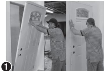
**1** Place bottom of door unit in bottom of opening. Lean top of door away from wall. Have helper caulk bottom of sill. Stand door upright, centered in opening and against wall.
