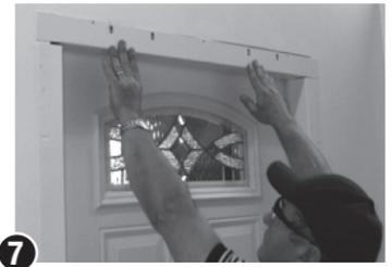
**7** Slide header closure trim into header. Adjust vertical and header closure trims for a good fit in top corners.
